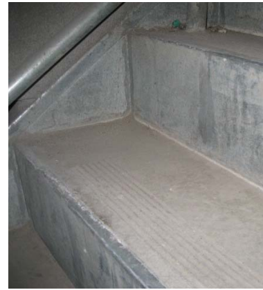
Figure 5: Metal risers in fire escape stair
