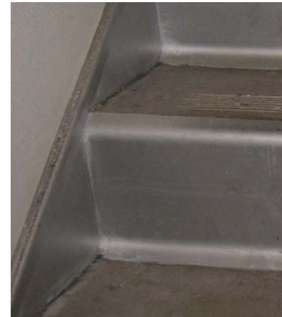
Figure 2: Radiused tread edge and tread-riser junction
